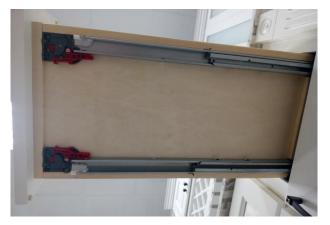
Step 7: Screw Slide into Cabinet Side Panels using preset center punch marks
