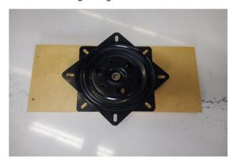
Step 2: Place Lazy Susan Berings on Tray with 2 of 4 screw holes showing and attach
