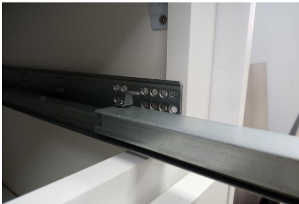
Step 8: Screw Slide into Face Frame
