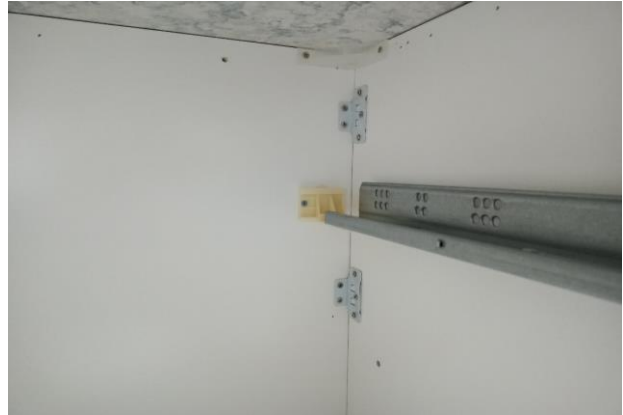
Step 7: Attach Rear Slide Clips to Cabinet and free floating Slide to Rear Slide Clips
