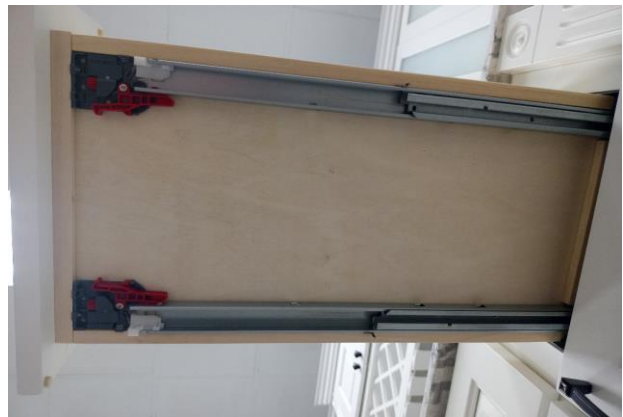
Step 9: Extend Slides and attach Drawer - Drawer will click into place when closing
