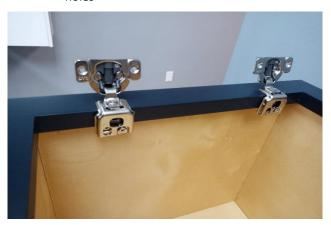
Step 8: Attach doors to hinges using #4 –  $\frac{1}{2}$ " Flat Head Screws in the 8 pre-punched holes
